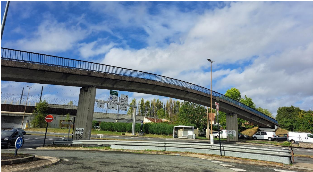
Figure 1 - Photo de la passerelle
